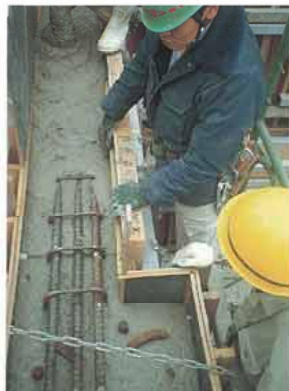
施工風景/Placing Super-workable Concrete
