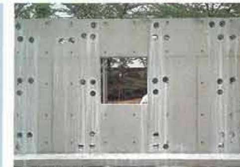
コア採取状況/Sampling of Core Specimen
