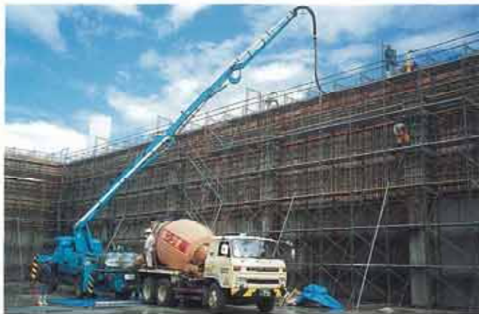
打設状況/Placing of Super-workable Concrete
