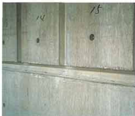
リブまわり充填状況/Surface of the Indented Ribs
